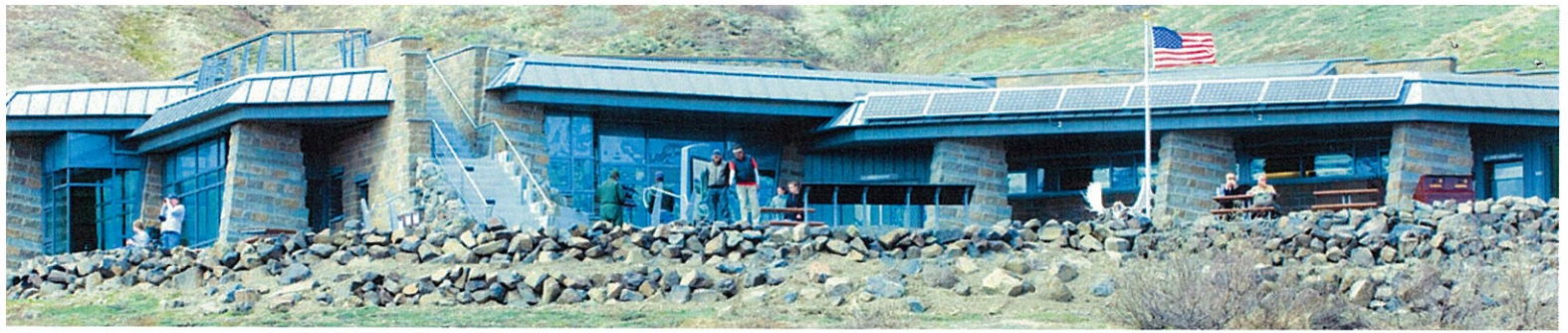
LEED Visitor Center, Denali National Park & Preserve, photo by Kent Miller
